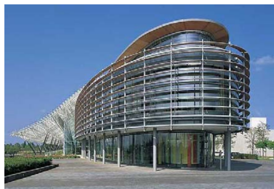
FinanzIT headquarters in Hanover, Germany (source: FinanzIT)
